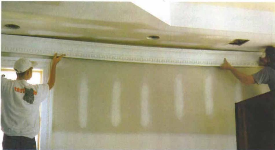
**Spring long pieces into place.** To make the seams disappear, butt sections are cut  $\frac{1}{4}$  in. long, glued up and sprung into place.
