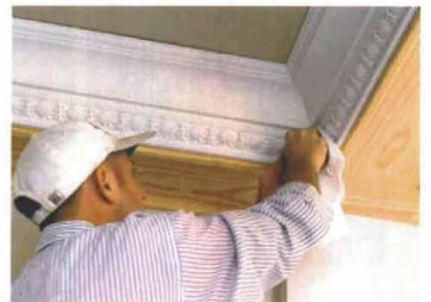
**A rag moistened with mineral spirits takes care of squeeze out.** Glue that gets on the face of the molding is wiped off before it sets up. Glue that squeezes out and dries can be scraped off with a knife.
