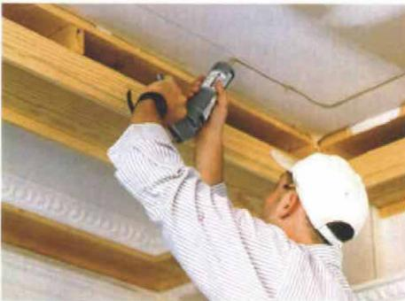
**Tracing lines for glue minimizes the mess.** A crew member runs out full-length  $\frac{1}{4}$ -in. beads of adhesive just inside pencil lines that denote top and bottom edges of the molding.
