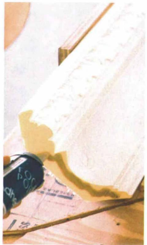
**Adhesive makes it permanent.** After dry-fitting the miter cuts in the setup jig, a  $\frac{1}{4}$ -in. bead of proprietary adhesive (see p. 120) is applied to each side of the joint.
