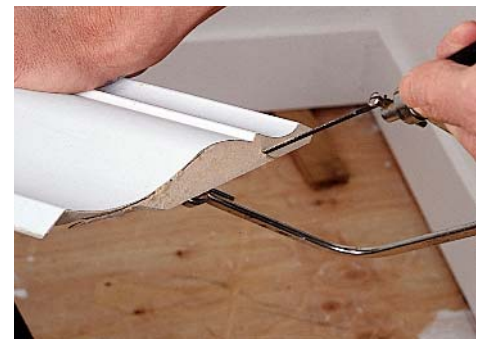
For best results, approach the cut from more than one direction.
