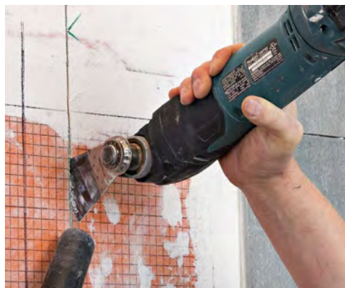
Cut the wallboard. An oscillating multitool makes short work of wallboard cuts, and a vac hose tames the dust.
