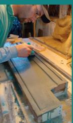
Give the texture some tooth. A slippery sill isn't safe, so I added a little texture with an old paintbrush while the mix was still curing. The brush also helped to smooth any surface imperfections.
