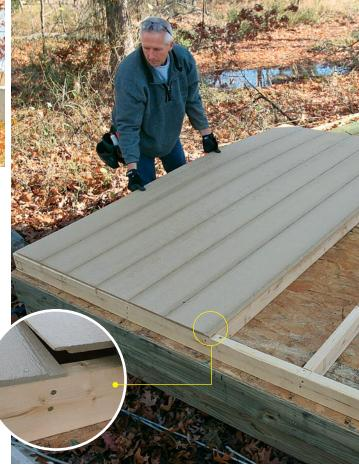
Let the walls lean out and the siding hang down. Once the wall is up, I brace it leaning out so that I can easily build and stand the gable walls on the floor deck. The 7-ft.-5-in. wall height allows the siding to hang down past the floor framing and act as a drip edge.
