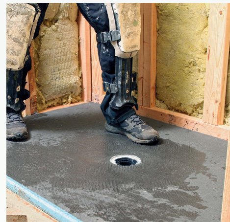
Place the pan. Walk all over the pan to collapse the thinset ridges and ensure the pan is fully bonded.
