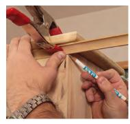
Attach the cove. Mark the cove sections using the case as a guide and fasten them with short brads and glue to the sides only. Fastening to the top could cause the cove to separate if the top expands from the heat.
