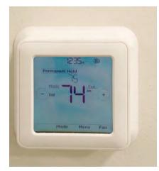
SIMPLE SYSTEMS ARE STILL SMART Basic Honeywell thermostats are used in conjunction with high-performance ducted HVAC systems. Keeping technology simple for first-time homeowners demands intuitive heating and cooling controls.
