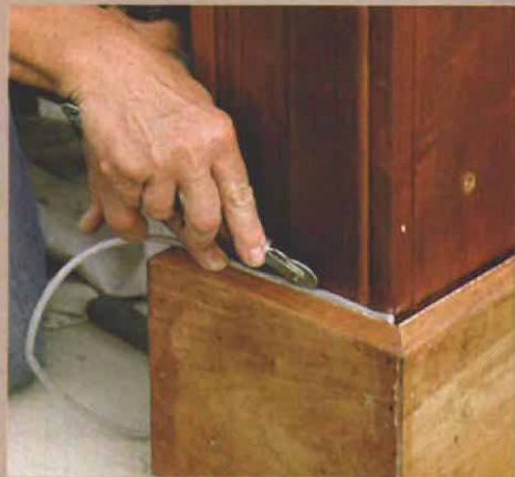
3. Backer rod allows caulk to flex.
