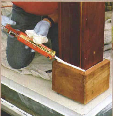
4. Polyurethane is the first line of defense.
