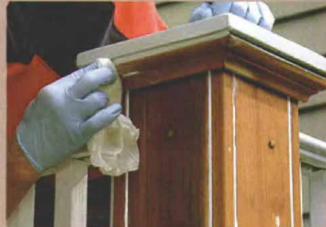
2. Mineral spirits remove excess caulk.
